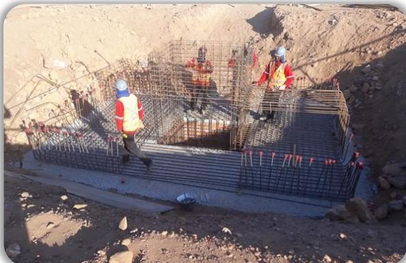
Execution of the 230kV substation's foundations
