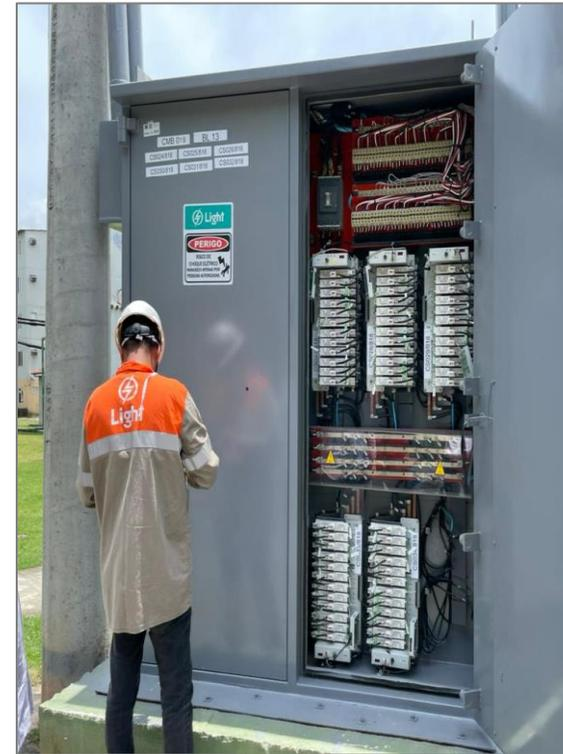
Loss-proofing measuring box for serving up to 144 customers
